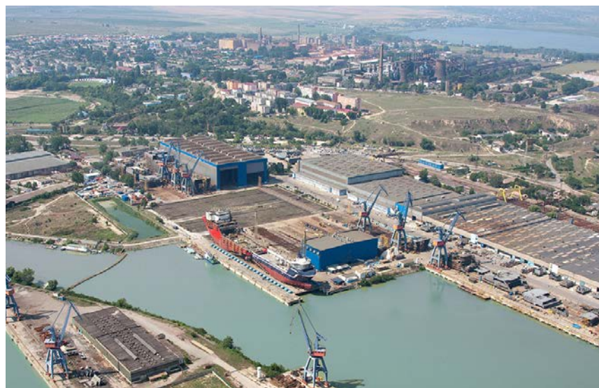
The krill ship’s hull will be made at Vard’s Tulcea yard in Romania.
